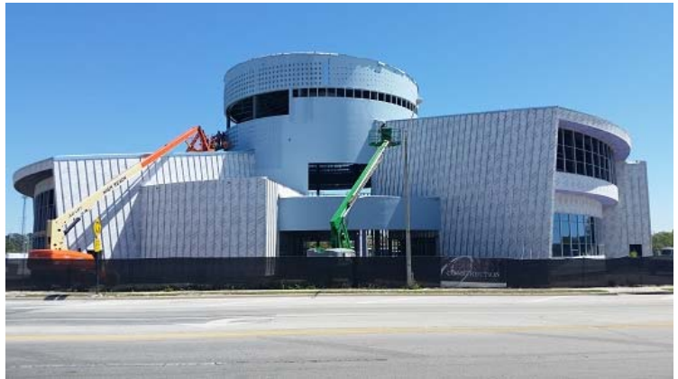
Photo by Central Florida Drywall & Plastering, Inc.
