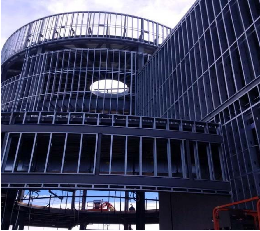
Photo by Central Florida Drywall & Plastering, Inc.
